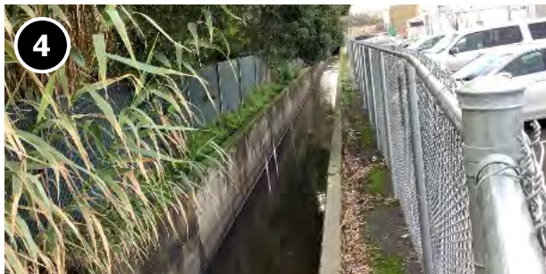
Channel adjacent to surface parking
