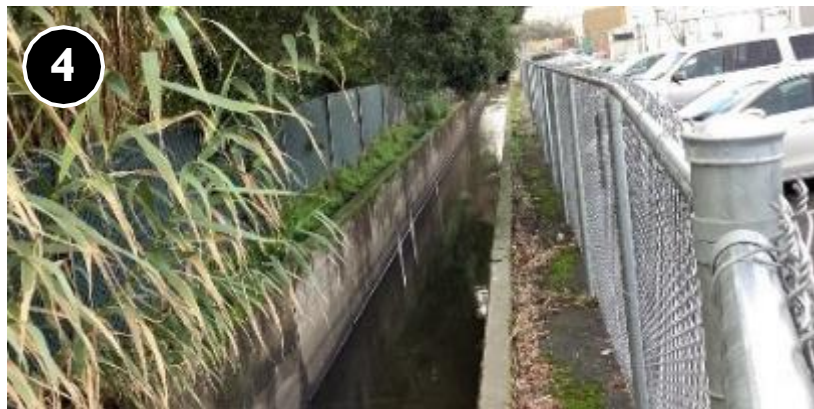
Channel adjacent to surface parking
